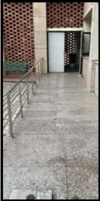
DIVYANG FRIENDLY ENTRY RAMP
